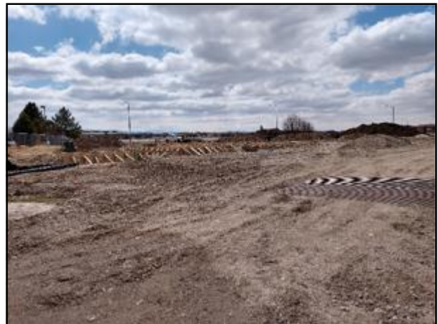
Groundbreaking has begun at Wheat Drive site
